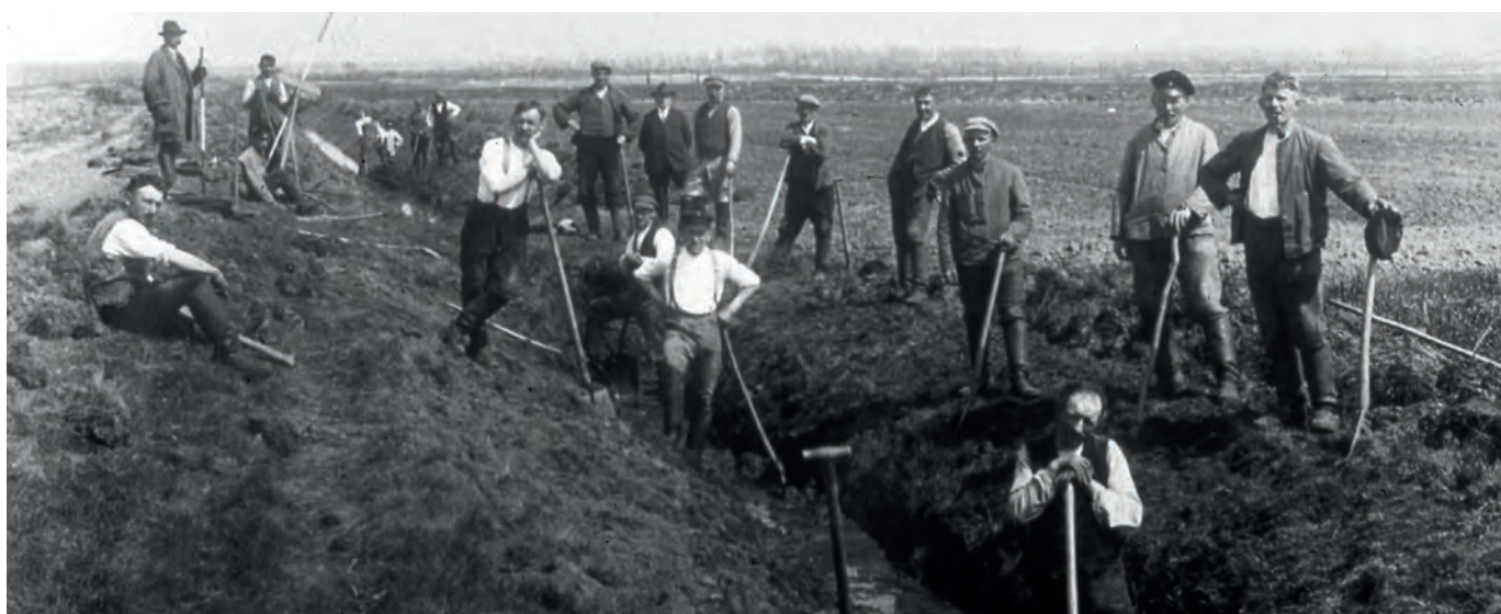
Figure 10: Ditch diggers during melioration in the Drömling in the 1920s.
